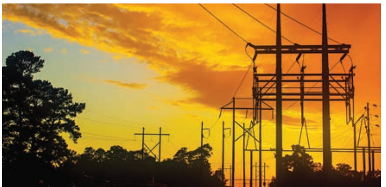
▼ MARK HUSFELD , Navasota Valley EC: Near a substation in Navasota after a thunderstorm.
